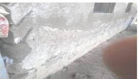
Fig. 2: Efflorescence on building at Gaa-Odota, Ilorin.
