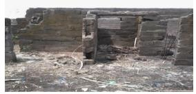
Fig. 4: Partial collapse of building at Gaa-Odota, Ilorin.
