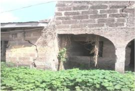
Fig. 7: Cracks on building at Gaa-Odota, Ilorin
