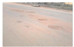
Fig. 8: Potholes on road pavement at Gaa-Odota, Ilorin
