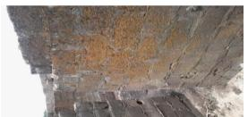
Fig. 3: Mold growth on building at Gaa-Odota, Ilorin
