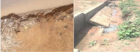
Fig. 9: Edge crack on road pavement at Gaa-Odota,Ilorin
